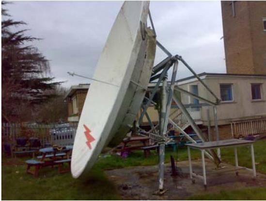
At the moment, the dish is configured for communications with geosynchronous satellites. This means that it is setup to point at a single static point in the sky. For the dish to be fully utilised, it needs to be adapted so that it can be steered and pointed in any direction.
