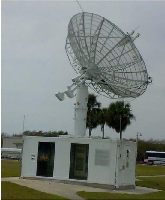
The upgrade of the dish to a fully steerable system should result in an installation similar to the photograph at the top of this page although this photograph shows a 7m mesh dish instead of the 5m solid dish that is available.
